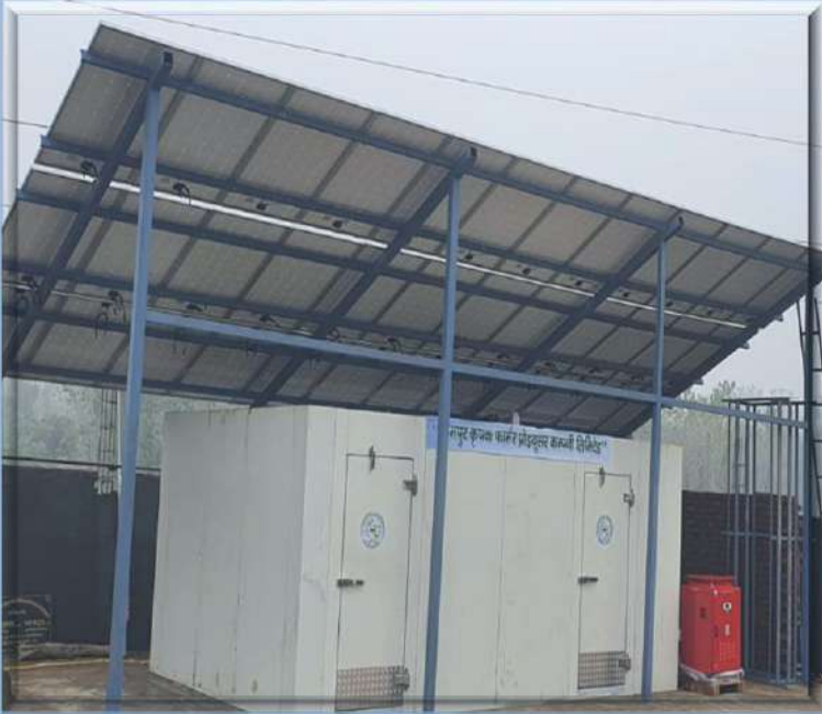
2 Solar Powered Cold Storage ,cap- 50 MT Farmer site Mob Solar Cap -6 MT by FPC
